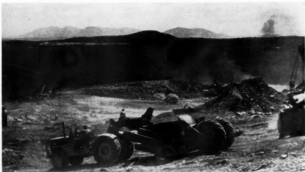
STRIPPING OPERATIONS AT RATTLESNAKE MINE IN UTAH.
